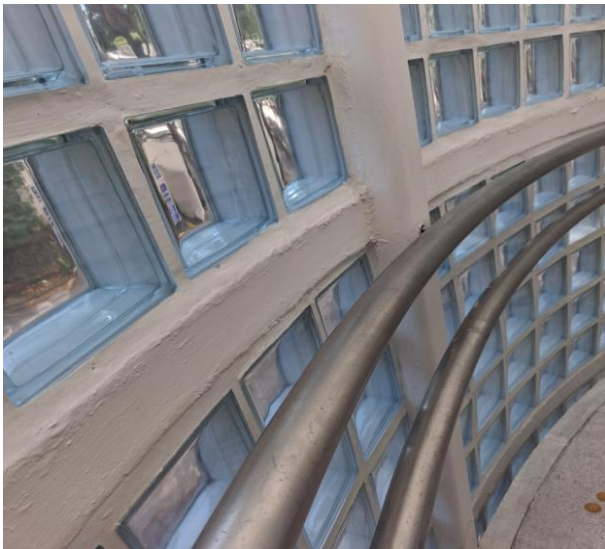
Above photo -External stair enclosed with cubicle glass wall, rigid not need aditonal support like curtain wall
